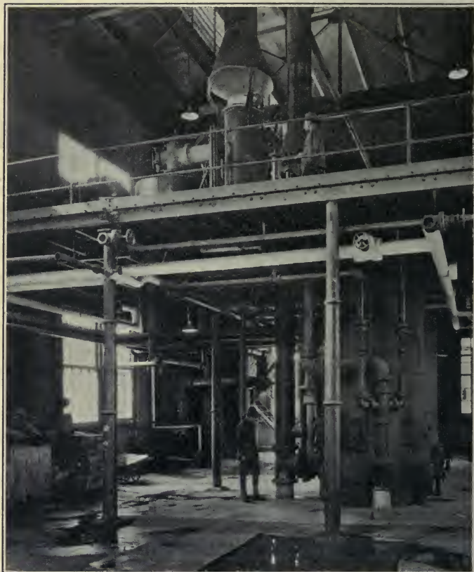
FIG. 23.—Furnace for Generating Carbon Monoxide.
